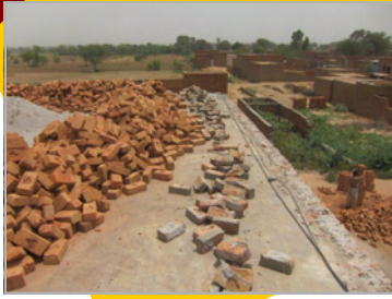
Pakistan shelter under construction
